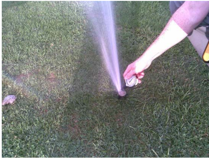
Fig 3. Measuring pressure at the nozzle using a pitot tube
